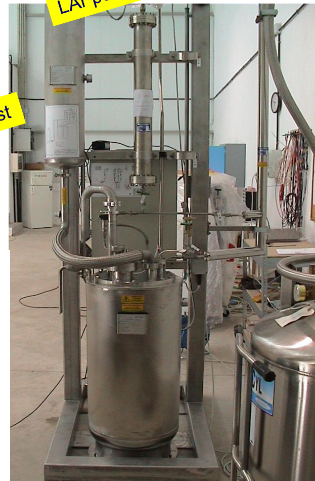
LAr purification station
